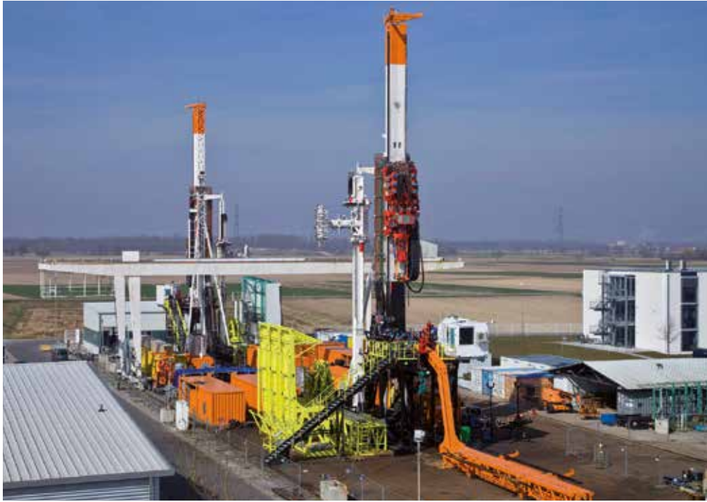
Deep drilling rig
