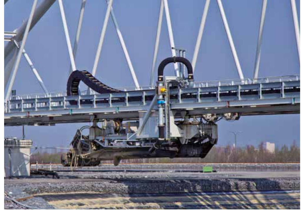
Sludge treatment plant
