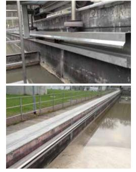
Longitudinal scraper, installed in the tank at Plauen sewage plant (Germany) Travel: 53m
