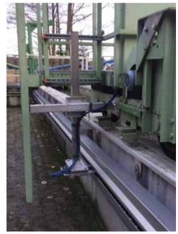
Sand traps with telescopic moving end arm Travel: 19m
