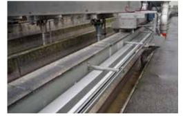
Sand traps: sewage plant in Bamberg (Germany) Travel: 26m
